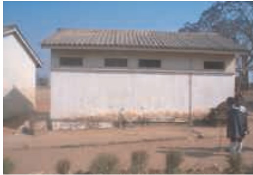
Disused toilet block - Before
