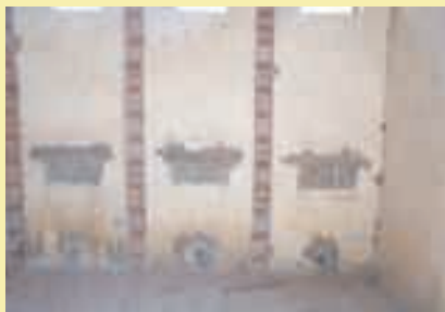
Internal alterations in progress
